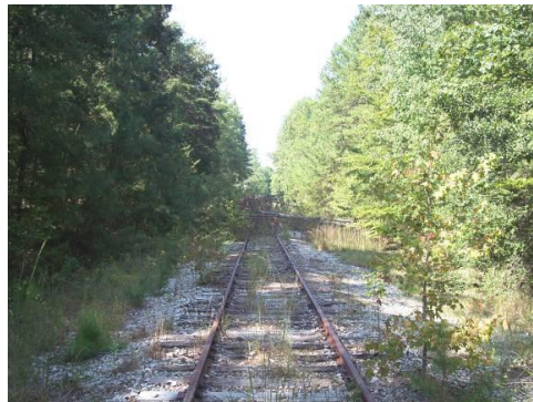
Greenville and Northern Rail Line near ICAR
