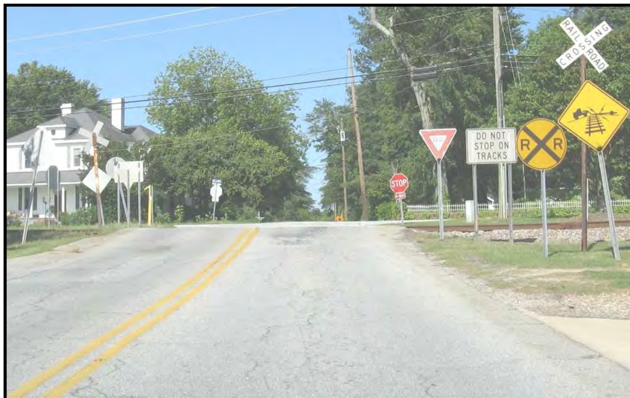
Figure 4-8: Richardson Street, Simpsonville, grade crossing with no protection
