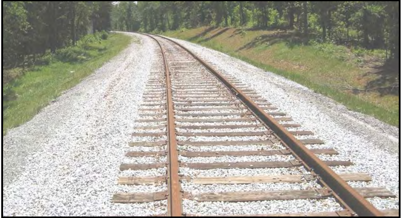
Figure 4-7: Track conditions at Woodruff Road in Greenville (excellent ballast and ties, rusty rail)
