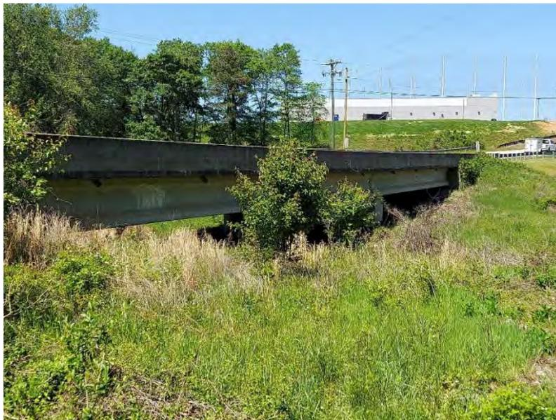
The Garlington Road bridge over Rocky Creek was constructed in 2006. The bridge is 160 feet long with 20-foot approach slabs and has a width of 39.25 feet with 36 feet of clear roadway. The cross slope of the bridge is 4.97%.
