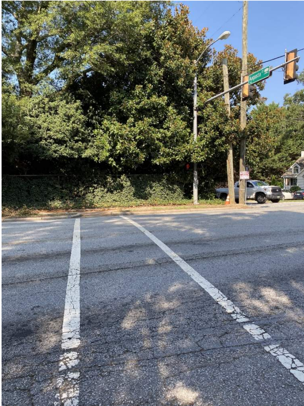
Signalized Crosswalk at Augusta Court
