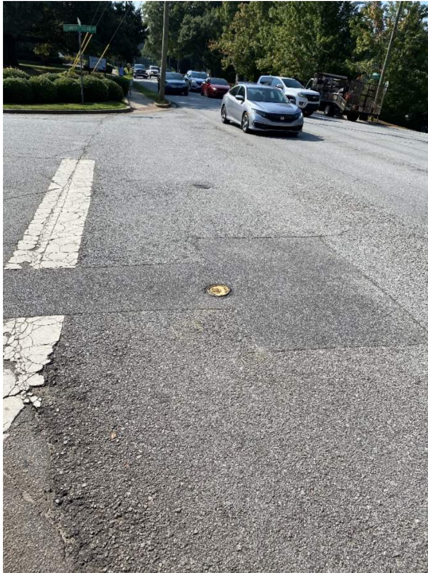
Missing crosswalk at County Club Drive.
