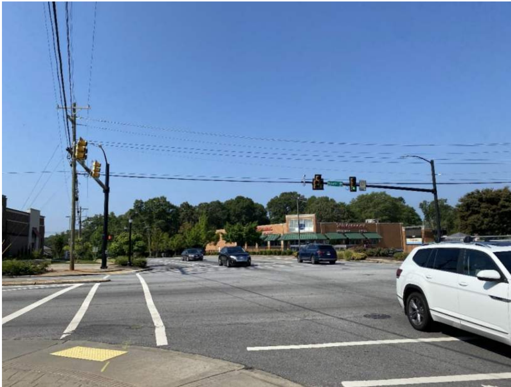
Existing Faris Road signal heads without retroreflective backplates.
