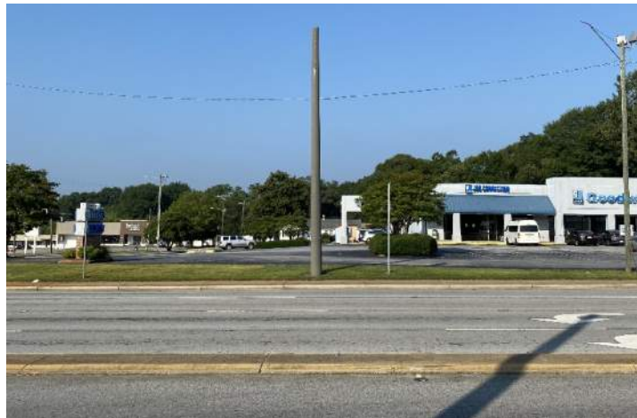
Obsolete Concrete Pole
